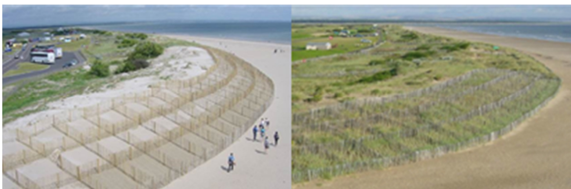
Figure 14.1 Soft engineering at West Links, St Andrews.
